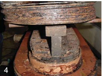
Above: (1) Lead failure and evidence of the resulting corona (2) Failure of copper turn (3) Damaged pole laminations (4) Deterioration of turn insulation
